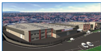
NEW PRODUCTION FACILITIES 2018 Scanzorosciate (BG)
